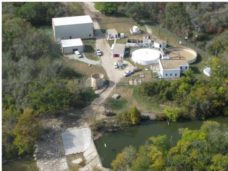
Photograph 2. Water Treatment Plant on Navasota River with City Dam
