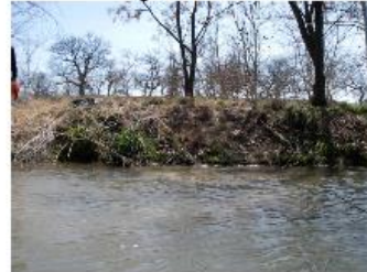
Right Bank View
