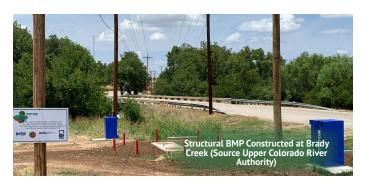
The installation will capture stormwater flows from a subbase of Brady Creek, route it to the vortex separator for treatment, and discharge the treated stormwater into Brady Creek. Two automatic
