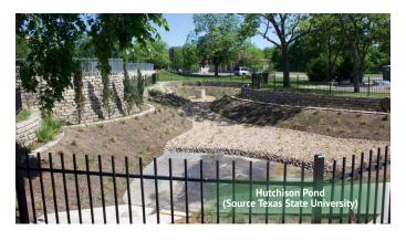
The Hutchison biofiltration pond is highly visible to the public as it is located near a popular river access point and receives runoff from downtown San Marcos. The pond was constructed using engineered soils and native plants that filter out pollutants from runoff. Once treated, the storm water runoff flows through an underdrain and into the San Marcos River. The estimated fiscal year 2020 load reductions from the Hogtrap retrofit and the Hutchison biofiltration pond are:
