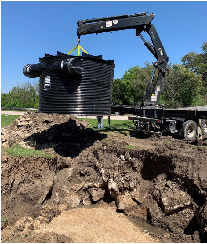
FIGURE 2.5 Installing the vortex separator (Photo by UCRA)
