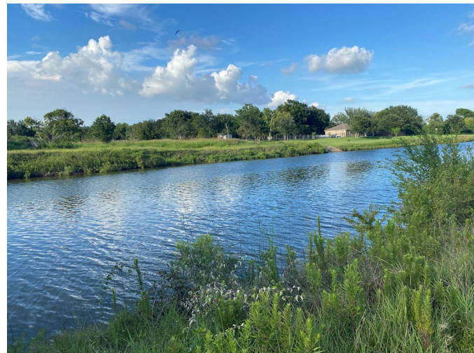
FIGURE 2.8 A section of Highland Bayou Diversion Canal (Photo by GBEP)
