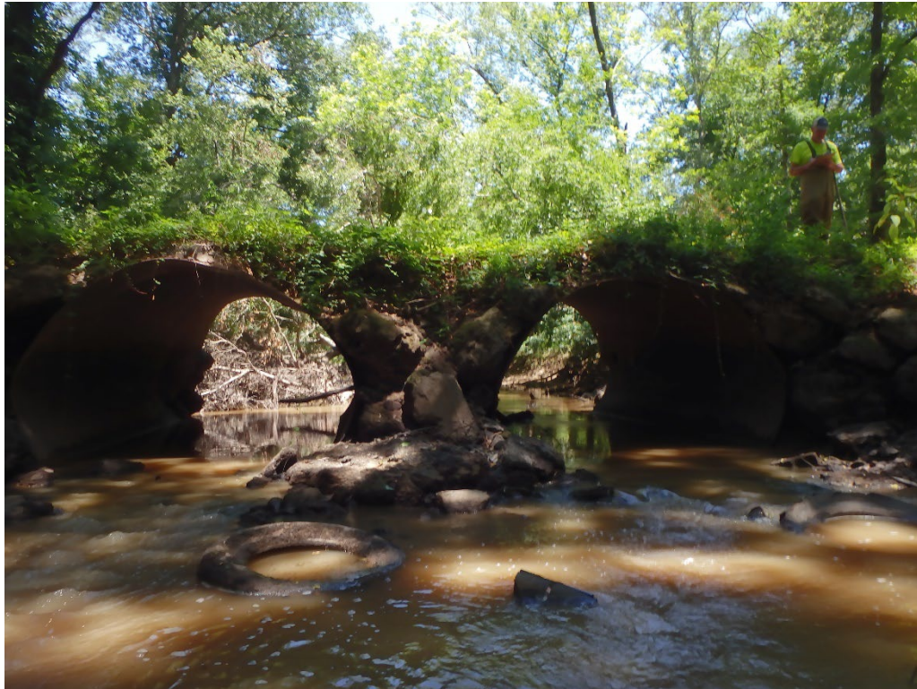
Figure 4.7 Photograph of Lilly Creek Site LC04 taken on June 22, 2021
