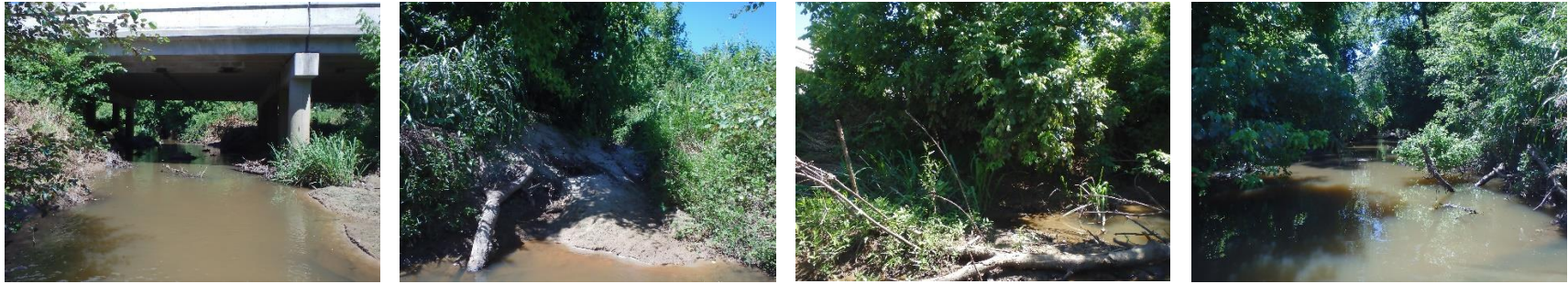
Photo group 5c: Site BC05; downstream, left bank, right bank, upstream. Taken on trip 1, 06/22/2021.
