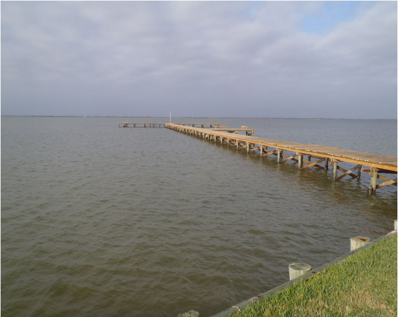
Carancahua Bay (Assessment Unit 2456_02; East side of Bay looking towards the West) near the intersection of CR 478 and CR 480
