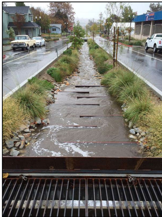
Figure 6. Photo of a “Slow the flow” initiative from the City of Paso Robles, California ( https://landarchs.com/award-winning-21st-street-turns-roadway-into-green-and-complete-street/ ).
