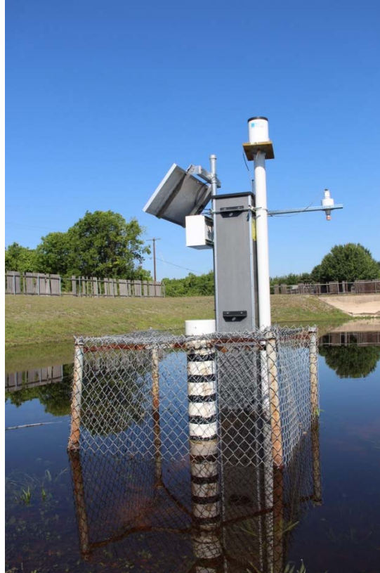
Figure 4. Valve Outlet Structure Installed at Pon Court Detention Basin.
