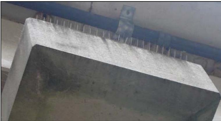
Figure 3: Pigeon Deterrents on Highway 16 Bridge
