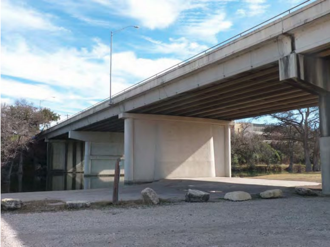
Figure 14. Final netting system over Spans 2,3, and 4 of Hwy 16 Bridge
