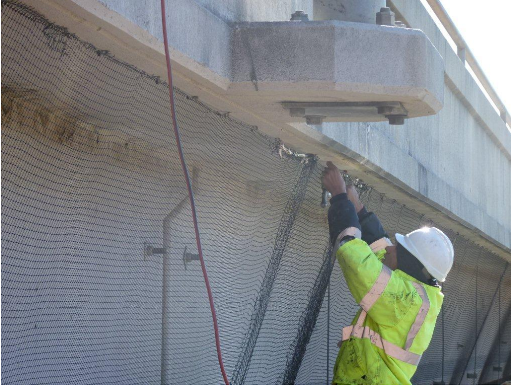
Figure 12. Installation of bird exclusion netting on Hwy 16 Bridge
