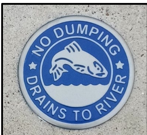
Figure 22. Storm drain marker installed in Kerrville
