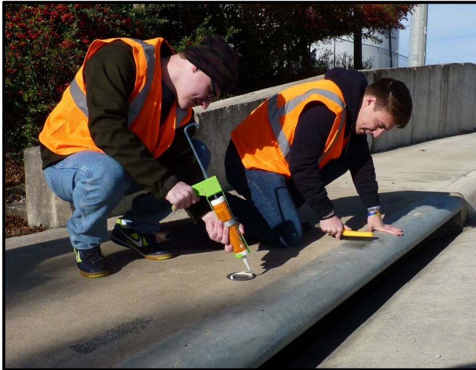
Figure 24. Installation of storm drain markers by Schreiner University students
