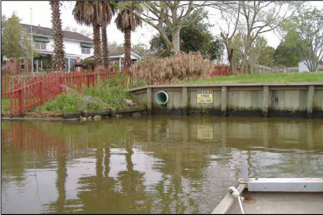
Figure 3-6 Typical Pipe, Clear Creek Tidal Area
