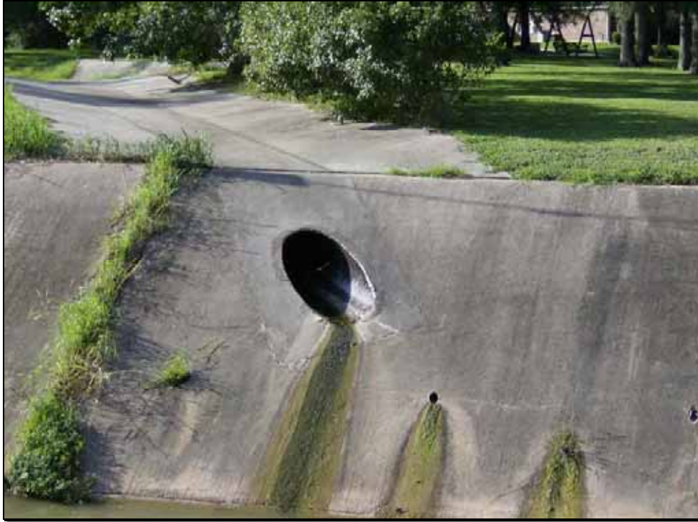
Figure 3-8 Typical Pipe, Mary's Creek
