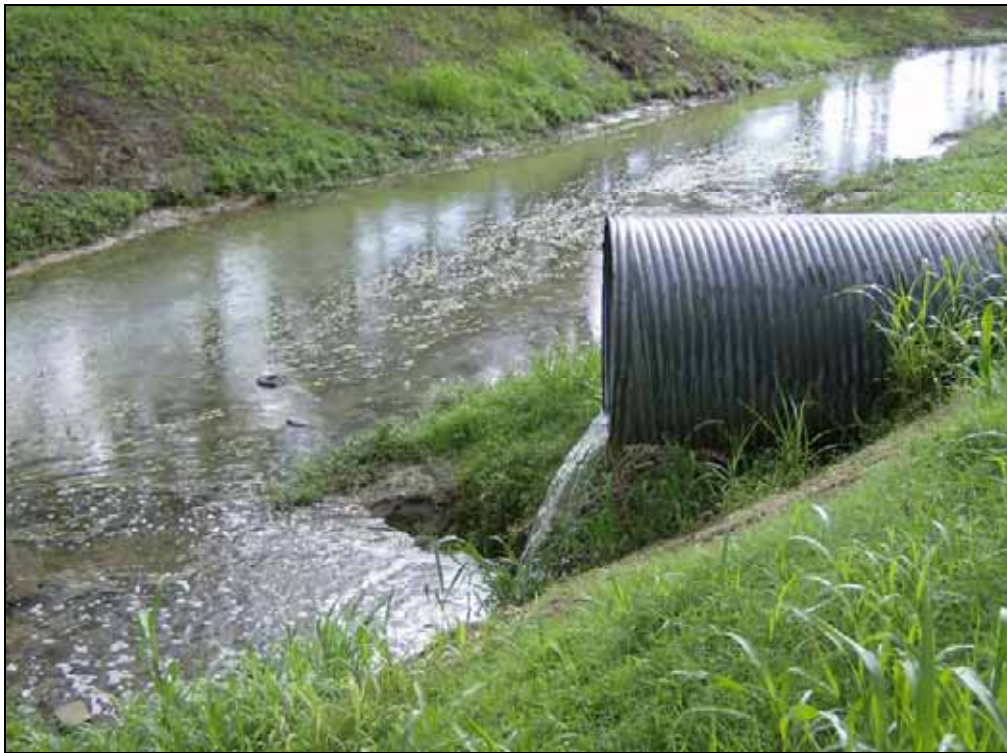
Figure 3-9 Typical Pipe, Mary's Creek
