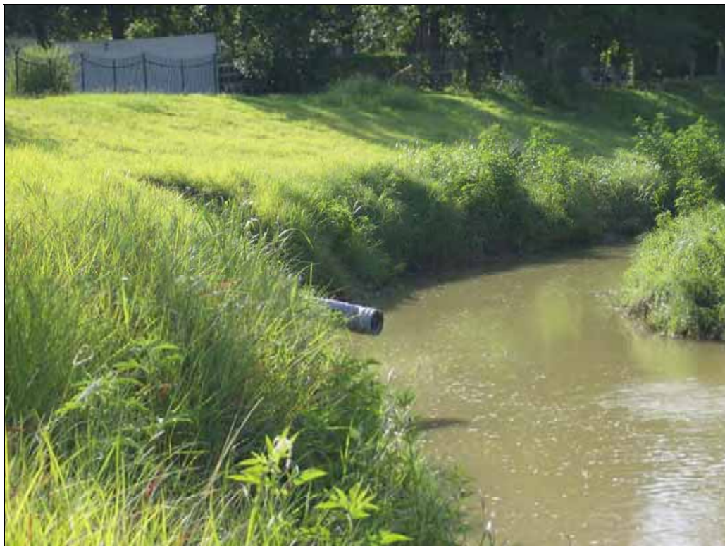
Figure 3-7 Typical Pipe, Mary's Creek
