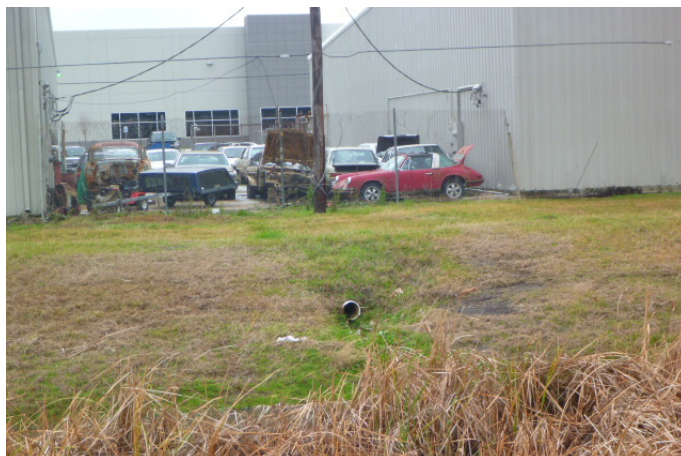
Figure 3-4: Example illicit discharge, Horsepen Bayou Tidal
