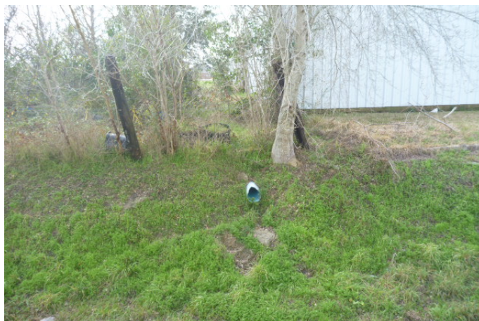
Figure 3-3: Example illicit discharge, Armand Bayou Above Tidal
