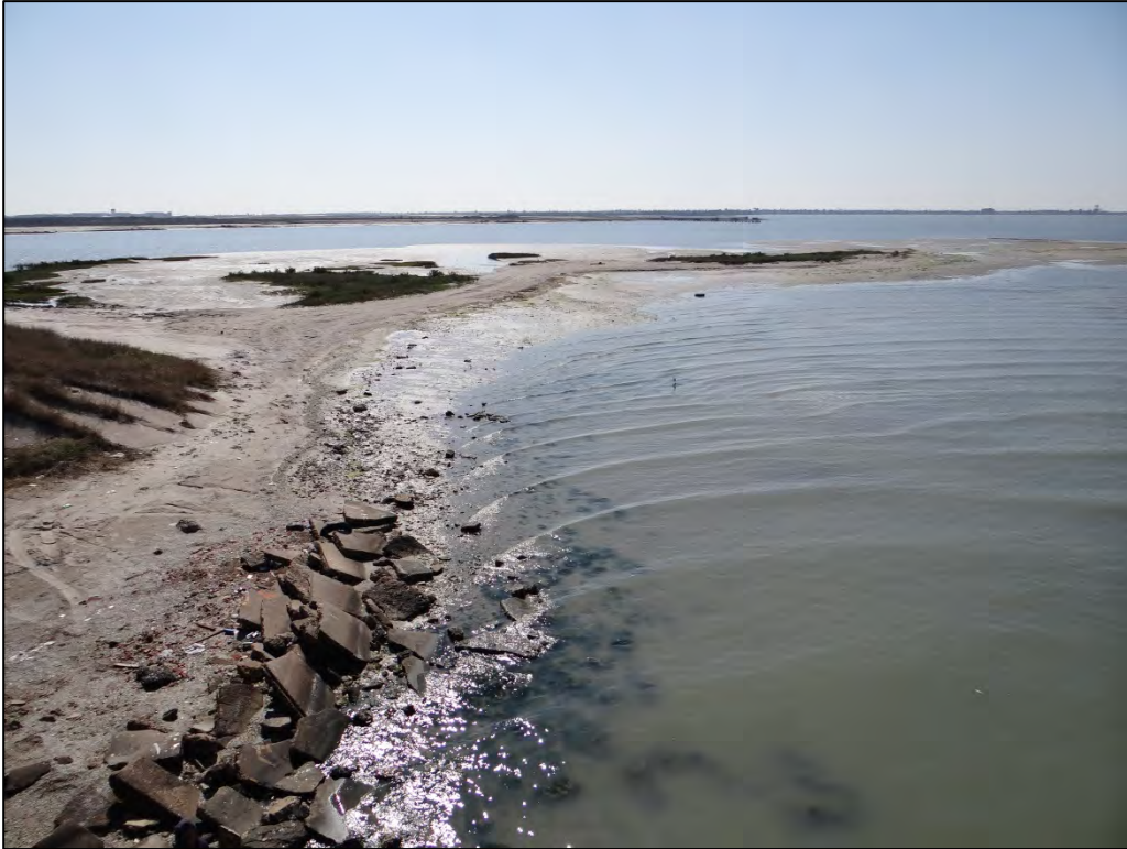
Figure 3.15. Station 13442 – Riprap along mostly bare shoreline.
