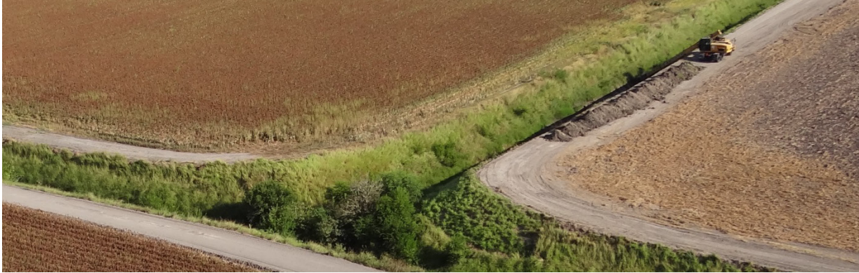
Ditch cleaning project on 2485C
