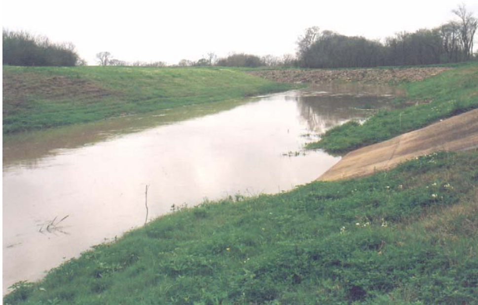
Station 12074, Flat Bank Creek at SH 6
