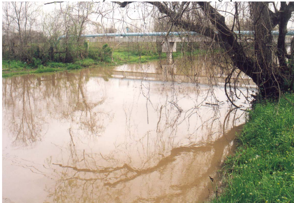
Station 12087, Oyster Creek at FM 1464 looking upstream
