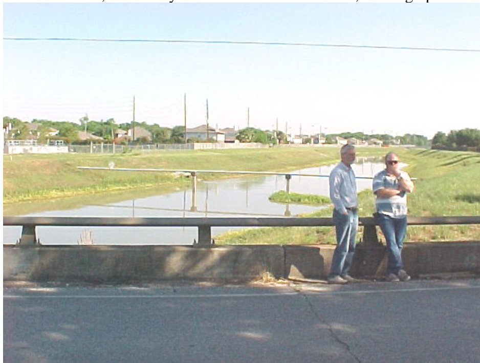
Station 11516, Red Gully at Richmond-Gaines Road, looking upstream
