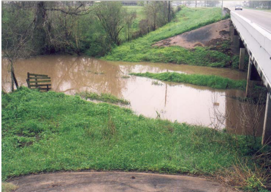
Photo 9: Station 12086, Oyster Creek at SH 6 looking downstream
