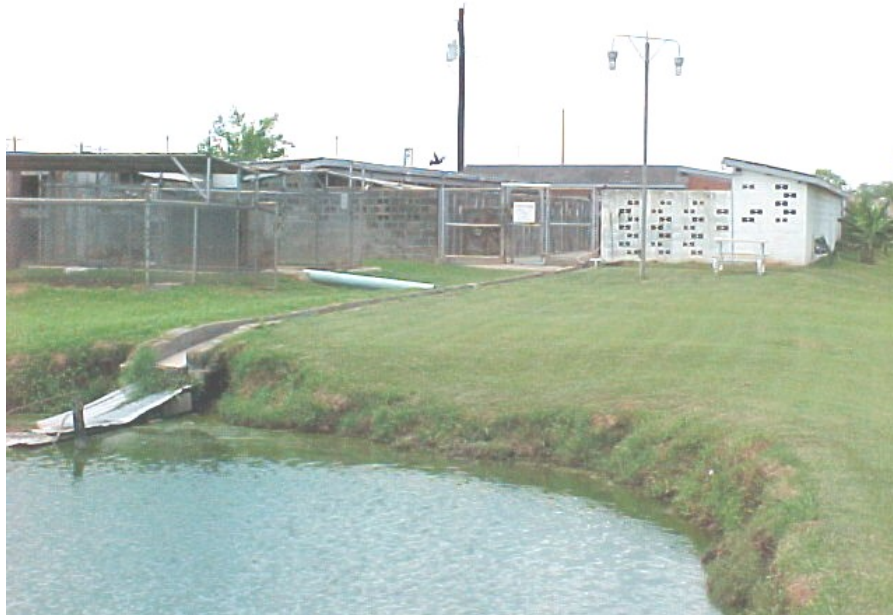
Photo 14: Drainage from the dog kennels waste lagoon at the TDCJ's Jester Unit
