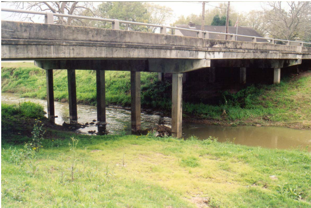
Photo 4: Station 17688, Stafford Run at El Dorado Boulevard
