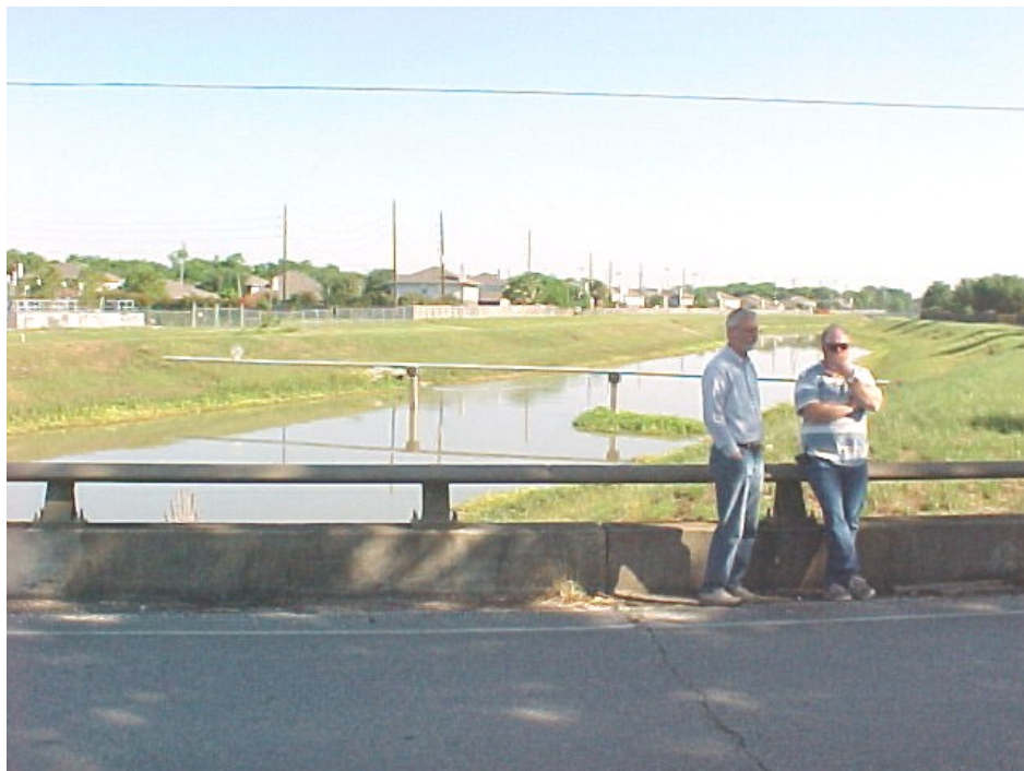
Photo 10: Station 11516, Red Gully at Richmond-Gaines Road
